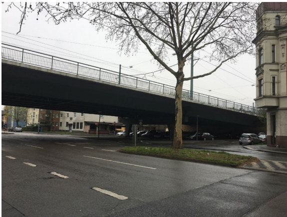
Figure 08 - Berliner Brücke saw from below (2019)
